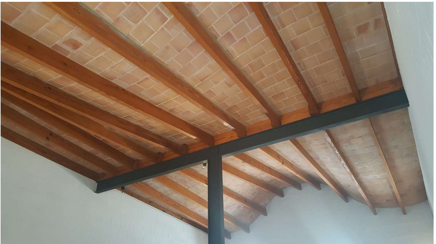
Sagrada Familia Schools sinusoidal bóvedas tabicadis with compressive concave inverting into adhesive convex (Antoni Gaudí, 1909).
