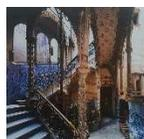
**Tradional Catalan stairs** supported one side, open in center, built by **escaleristas**, curve for **staircase vaults** by **hanging a chain** from supports, **inverting as formwork**.
