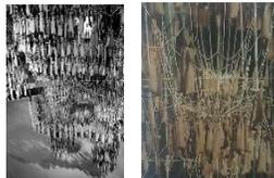
On arches, at **intersecting points**, where pillars would sit atop, **small canvas bag filled with lead shots, proportionate to building weight applied** to arch by pillar. Likewise, the pillars supporting the arch below, tied off at that point.
