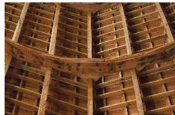
**Parabolic arcs** of **short timbers bolted end to end, as worker bees linked together.**
