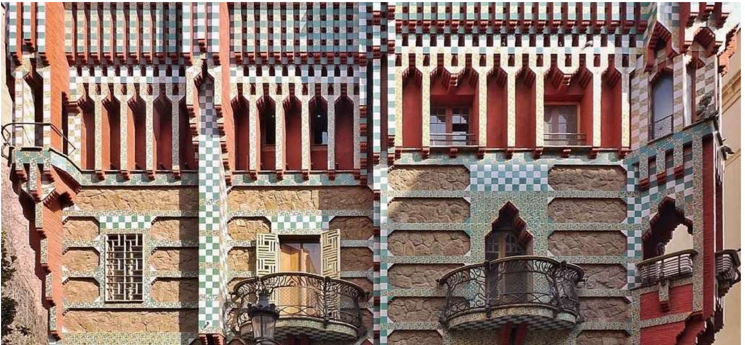
Parataxis of materials, textures, colors, exposing structural stone as finish material tracery pattern plate within Mudejar decorative border frame, made of serially produced industrial materials and a single unique marigold tile (Casa Vicens, Antoni Gaudí, 1883-88).
