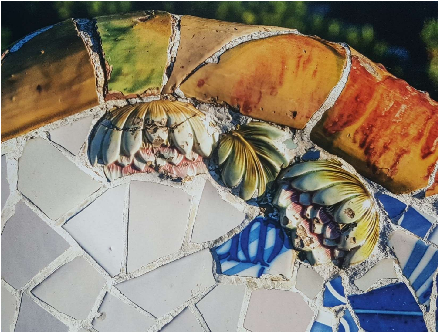
Trencadís Mosaics irregular shapes, economizing use of discarded materials laid by lesser skilled communal labor, adding color, energy, life by elevating broken pieces to beauty, through honest application and expression (Park Güell, Antoni Gaudí, 1910-14).
