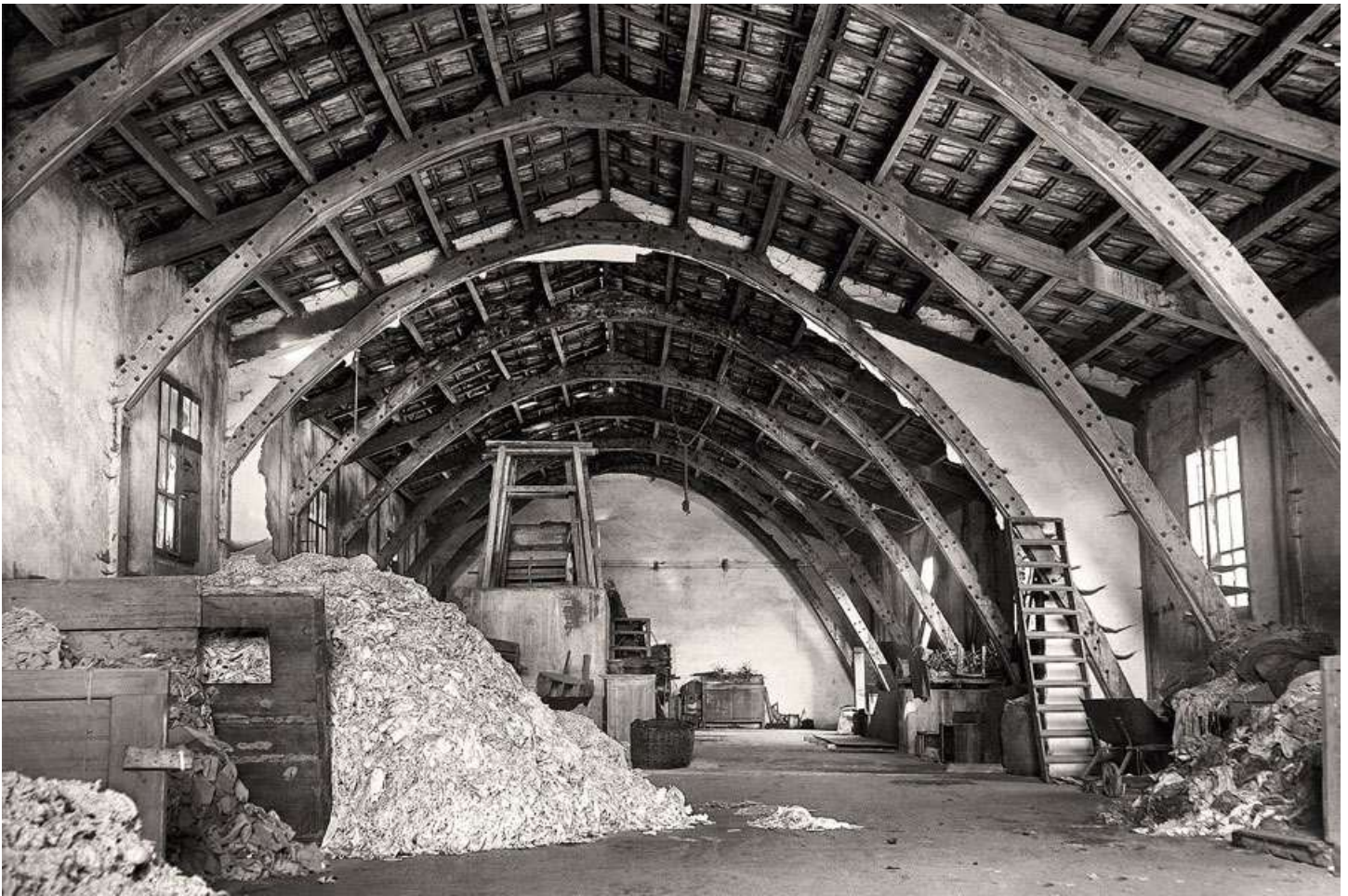
Wood beams bolted together into parabolic arches to provide open floor space within the cotton bleaching facility for the Mataró Workers Cooperative, of which Gaudí was a member and received his first building commission (1883).
