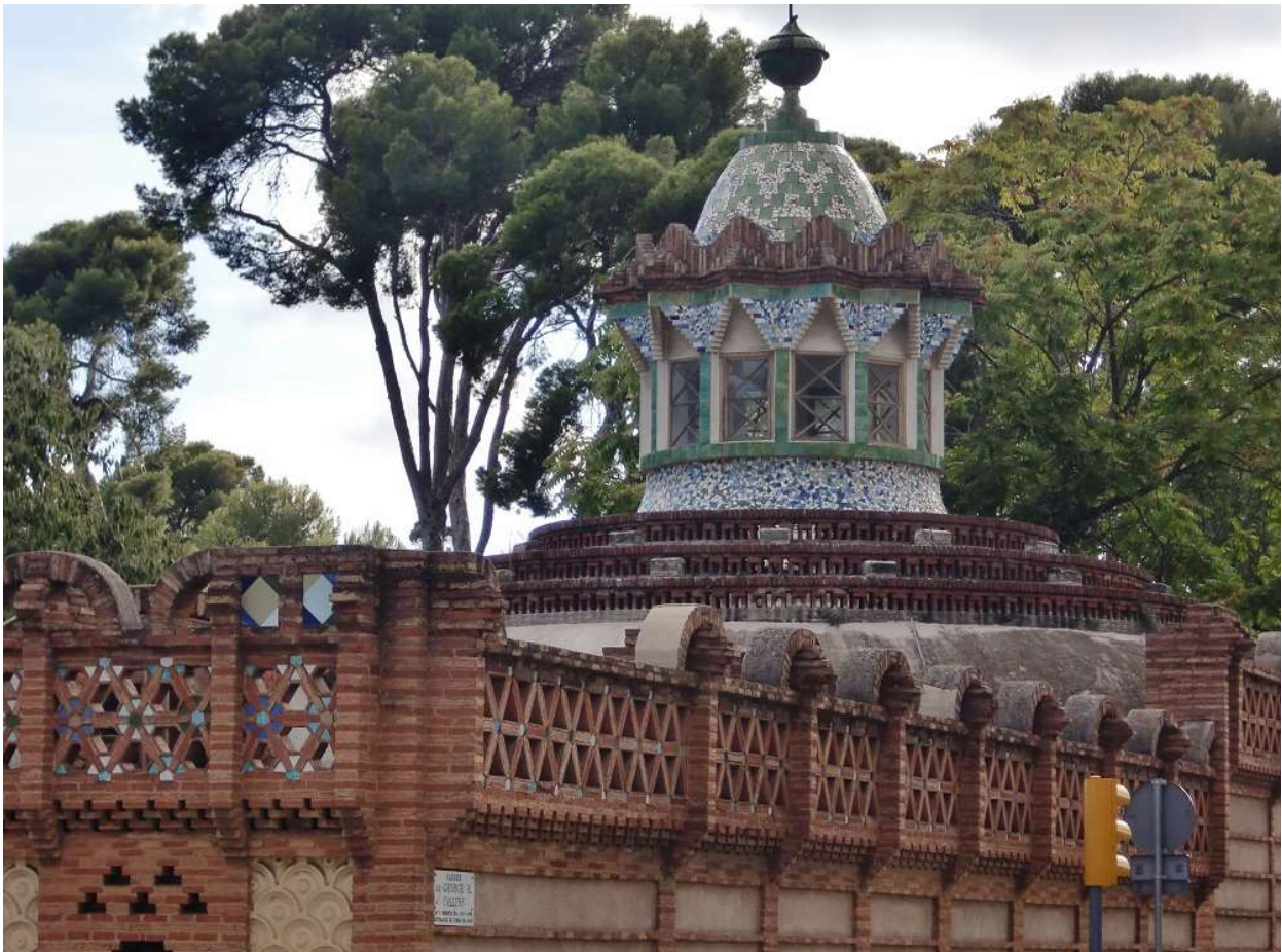
Pavellons Güell with trencadís mosaic infilled between standard tiles on lantern parabolic dome (1887).
